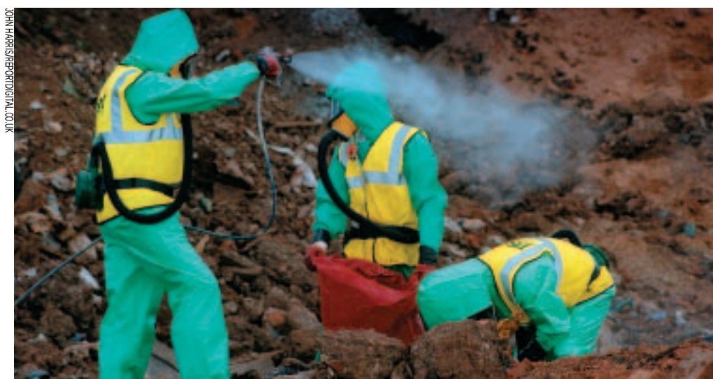
Contractors wearing protective clothing and breathing apparatus removing asbestos from a Stratford on Avon refuse tip. The asbestos was found by workers clearing the site for housing to be built. Nearby residents had been worried about the contents of the tip and the potential health risks for some time. Council officials and Health and Safety inspectors monitored the removal.
