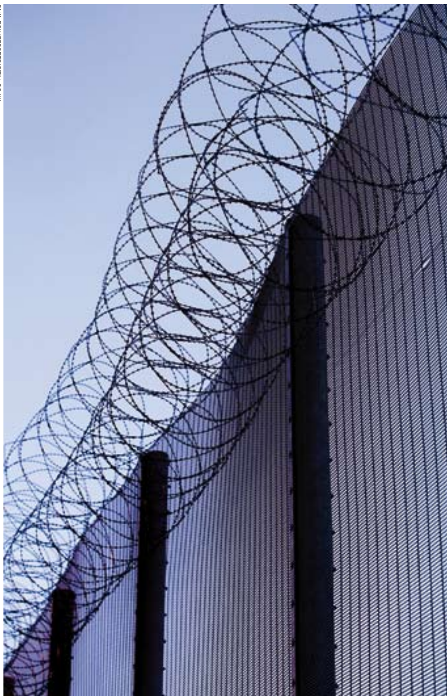
Razor wire fence for the Avon control centre building
