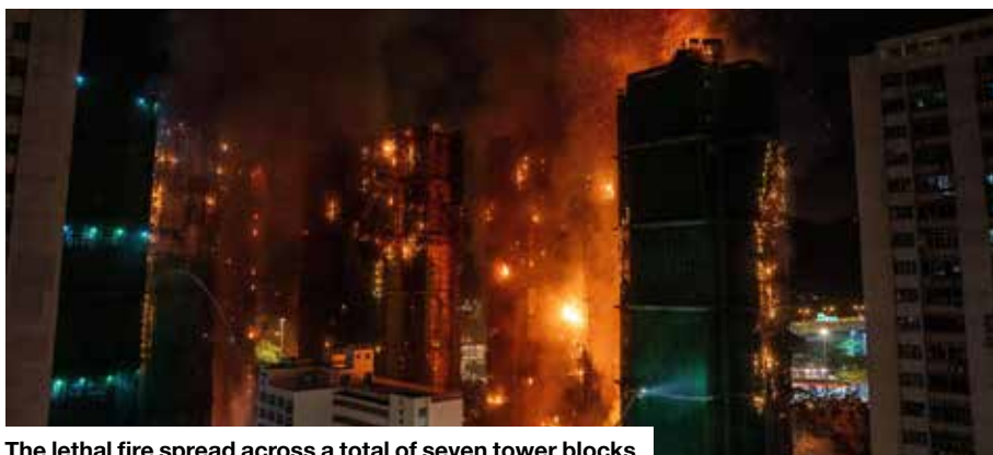
The lethal fire spread across a total of seven tower blocks
